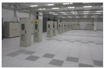
Most modern colocation facilities provide finished data center suites or secure cages with a raised-floor or slab whitespace — customers just need to install their cabinets and IT equipment.
